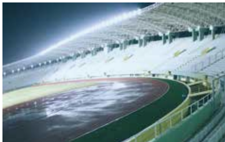
Éclairage installations sportives
